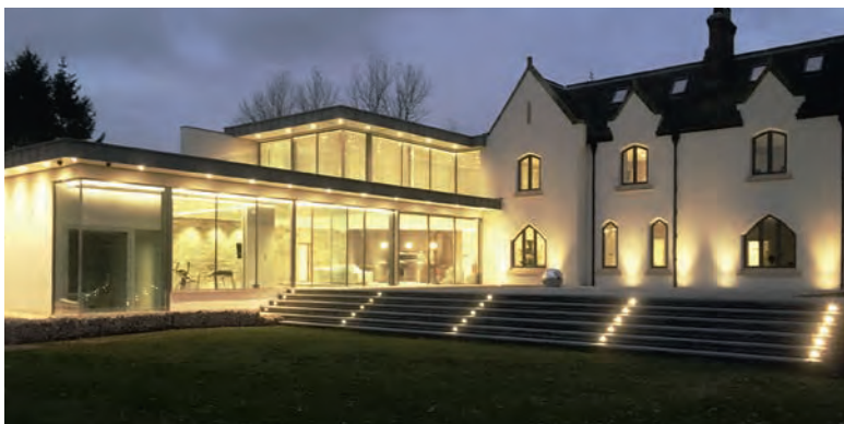
Above: The Logix system was used as part of a hybrid construction for this extension, in tandem with steel frame and swathes of glass. This allowed for a concrete upper floor structure and external balcony, whilst also offsetting the heat loss from the glazing. The 4m tall ground floor walls were cast in a single operation
